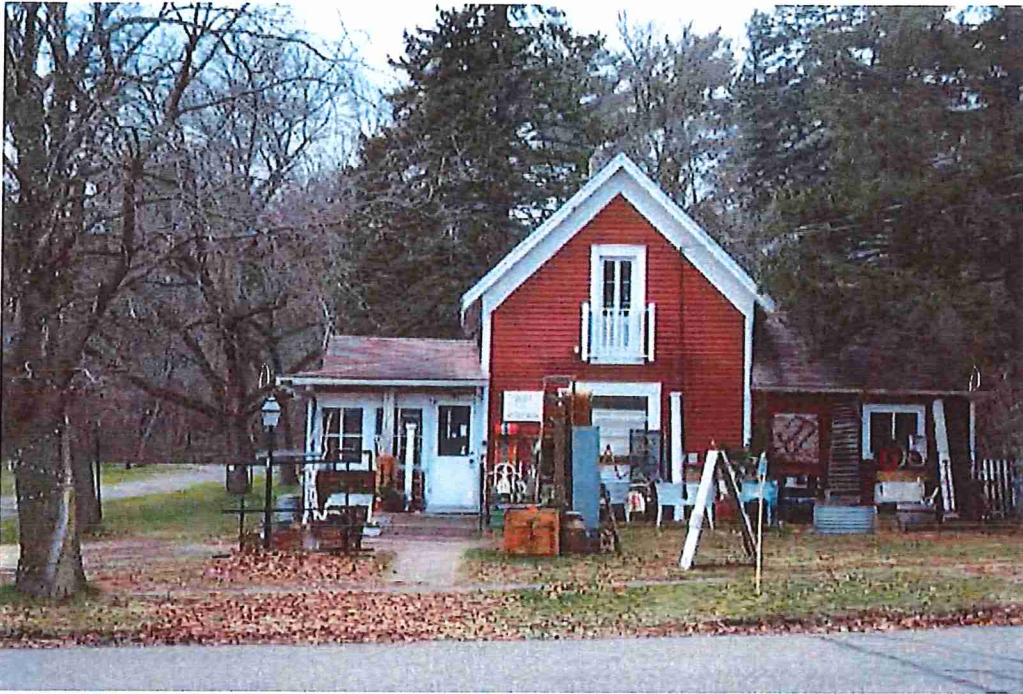
The porch to the south of the front gable elevation was once open but is now enclosed.
