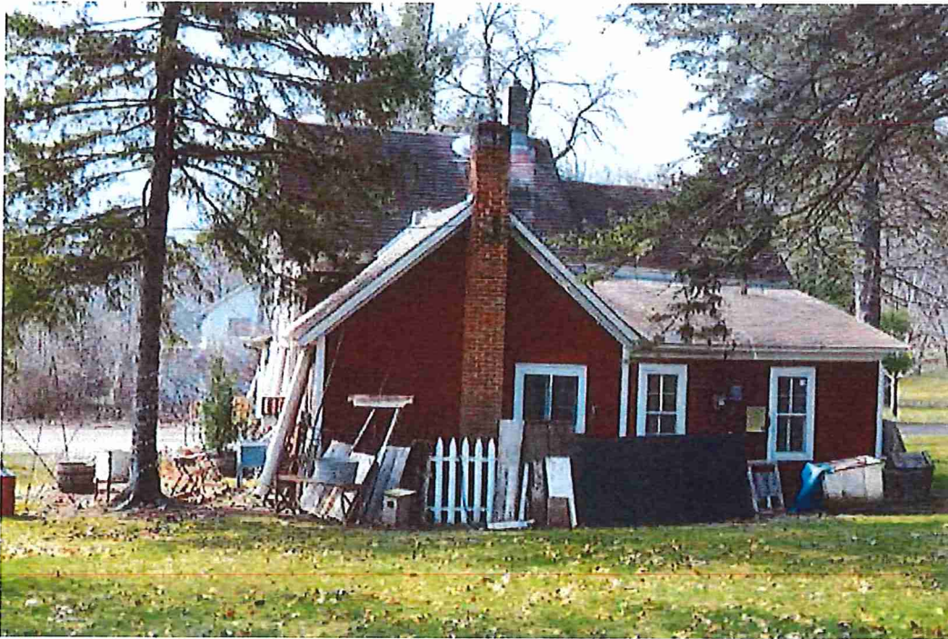
The north-facing elevation displays some of the cottage's complex growth of lean-tos and additions.
