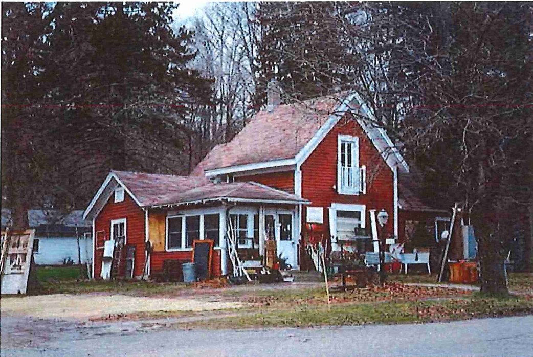
The Reverend Simon Putnam House sits on the northwest corner of the intersection of 32 nd Street South and St. Croix Trail South. Architecturally it is a folk cottage that has grown through time with additions to the north and west.
