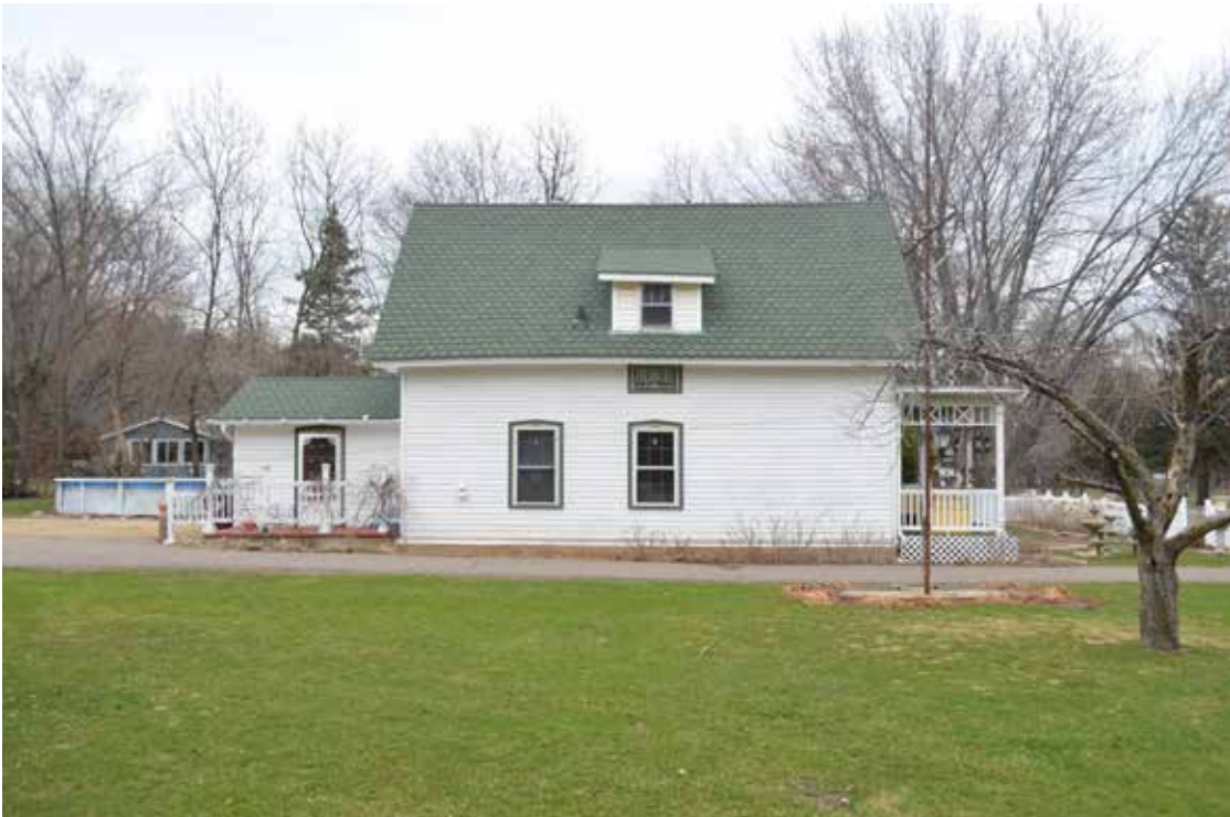
While it is difficult to determine what is original or modified on the south-facing elevation, it retains a simple balance of design.
