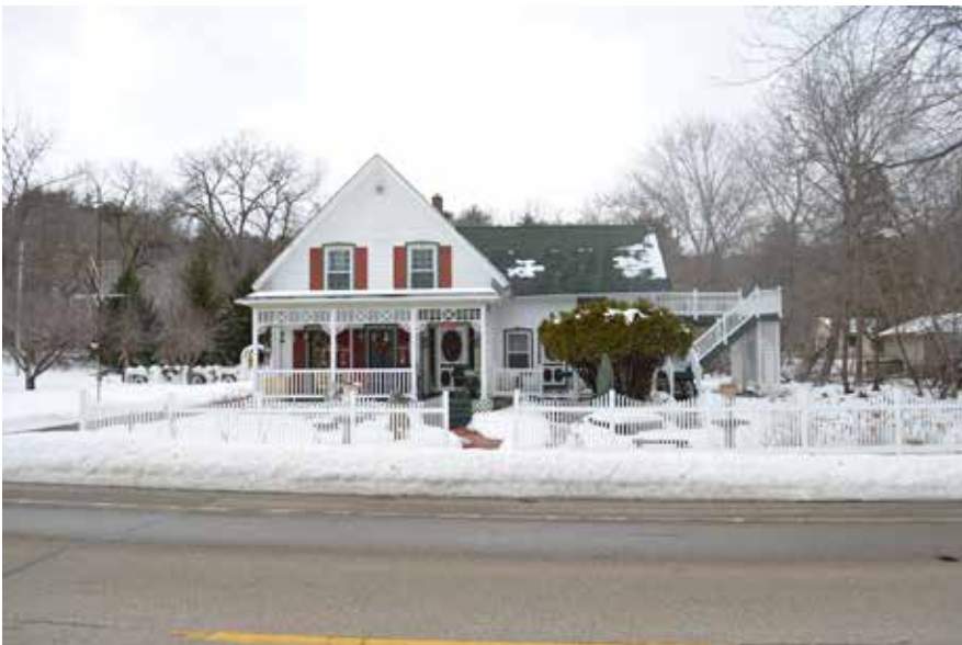
The Asa Tracy House has retained much of its original cottage feeling, but also been modified in many ways. The fenestration on most of the elevations has remained intact but the trimmings have been changed over time.
