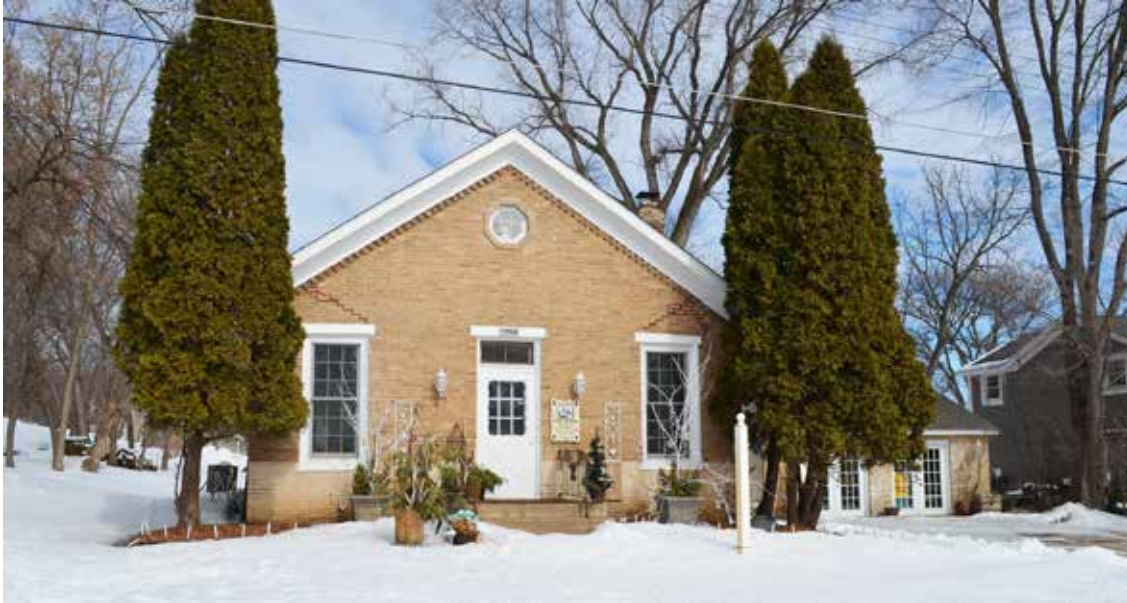
The Village School retains much of its original architectural profile. While it has lost its bell tower and an octagonal window has been added to the front façade, the brick detailing, fenestration openings and simple, rectangular footprint remain intact.
