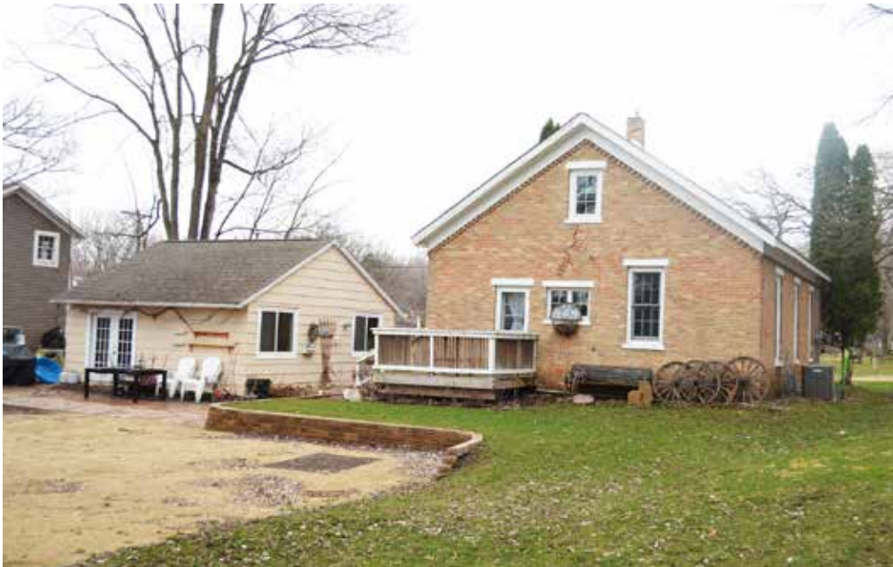
The north-facing elevation. Note that while the majority of the openings are original the divided light windows are newer, insulated windows.
