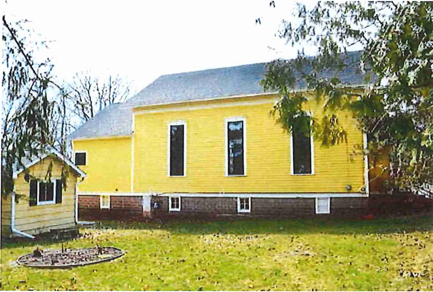
Looking to the south-southeast at the north-facing elevation with the later, lower-roofed addition to the back of the original simple rectilinear structure.
