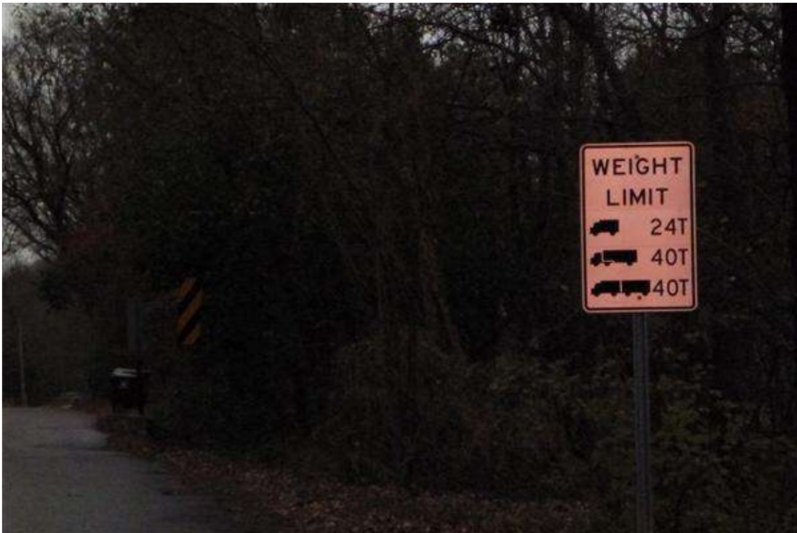
Photo 10 - recently installed load posting sign
