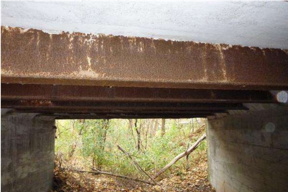
Photo 4 - steel beams looking north
