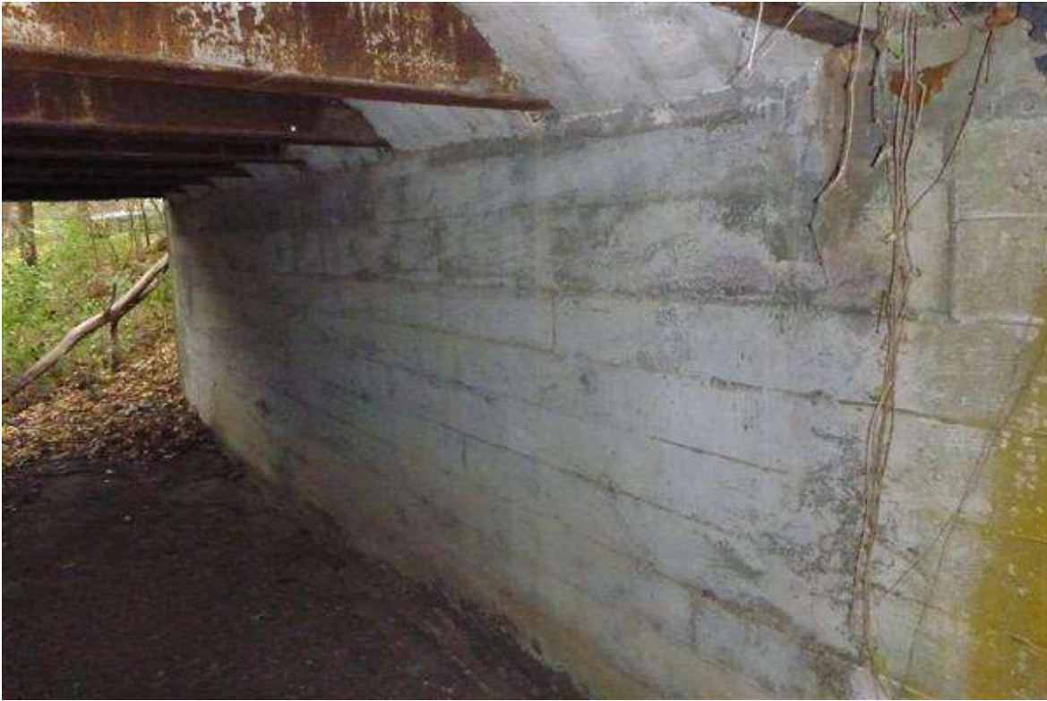
Photo 5 - west abutment looking southwest
