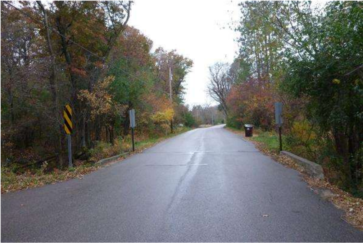
Photo 1 - Roadway over covert looking west
