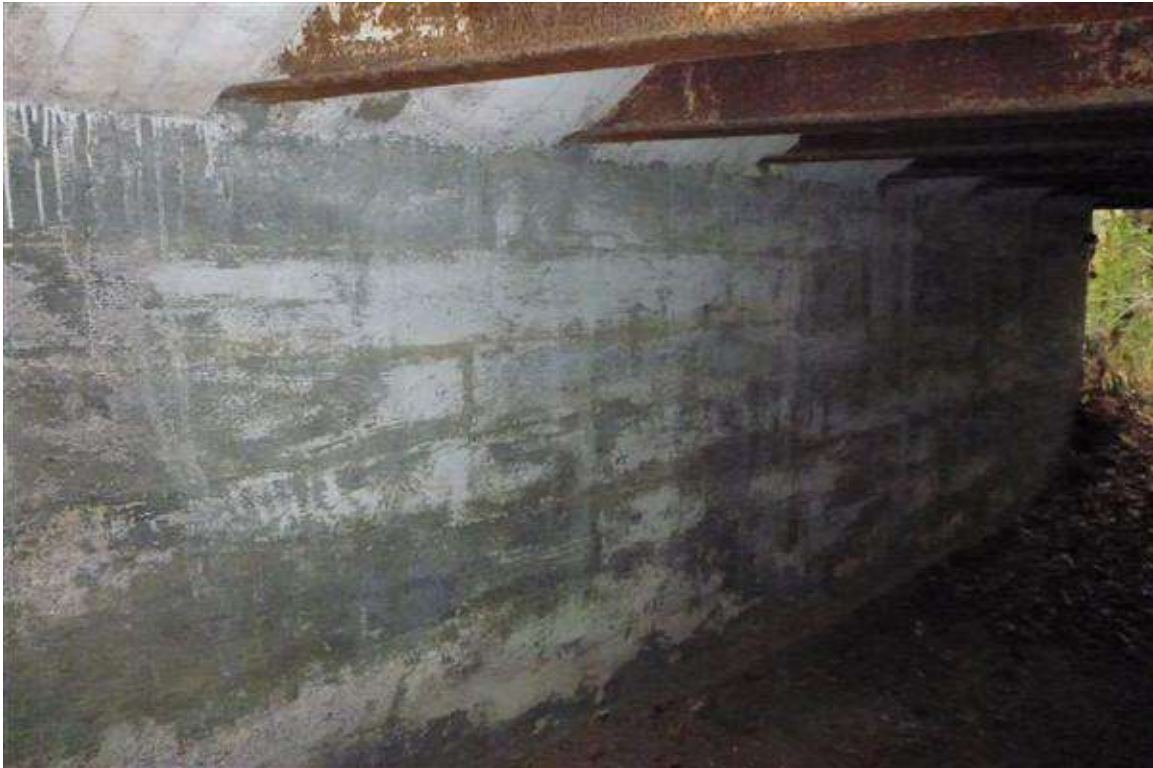
Photo 6 - East abutment looking southeast
