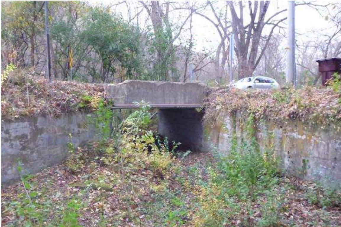
Photo 2 - upstream headwall looking north
