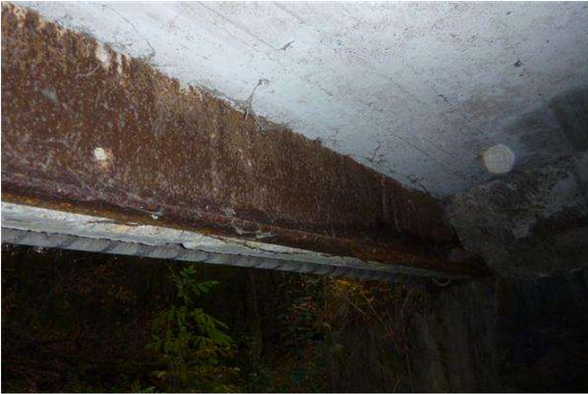
Photo 3 - south fascia beam looking south
