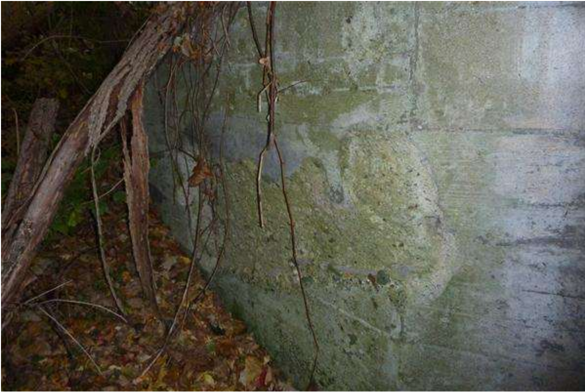
Photo 7 - north east wing wall
