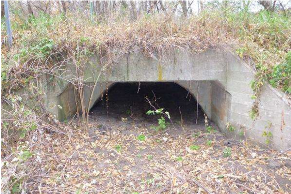
Photo 6 - east headwall looking west
