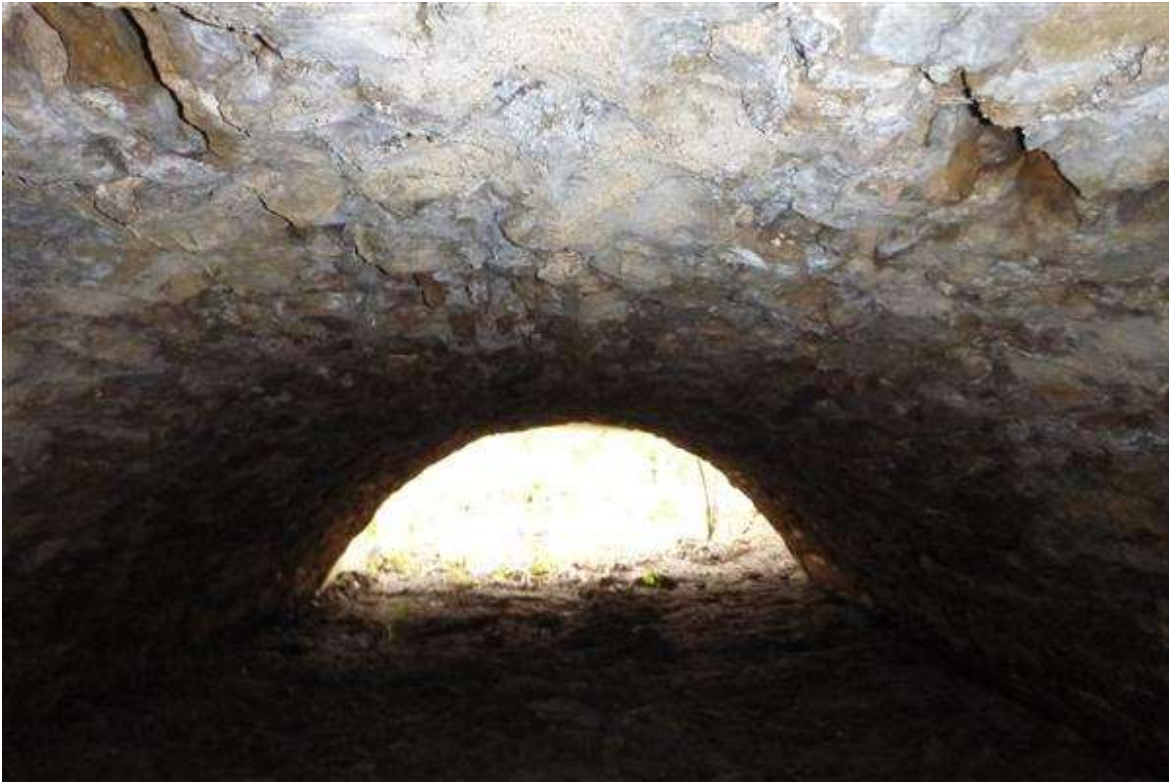
Photo 3 - masonry barrel looking east
