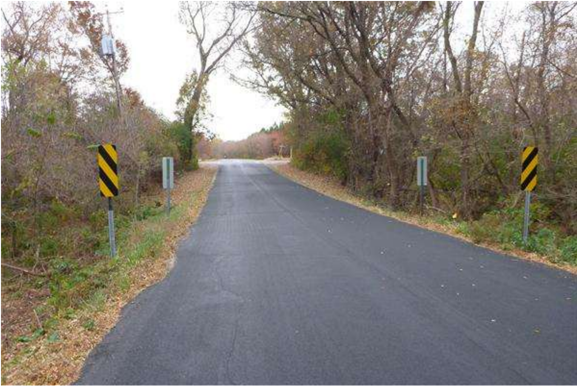
Photo 7 - Roadway over culvert looking south
