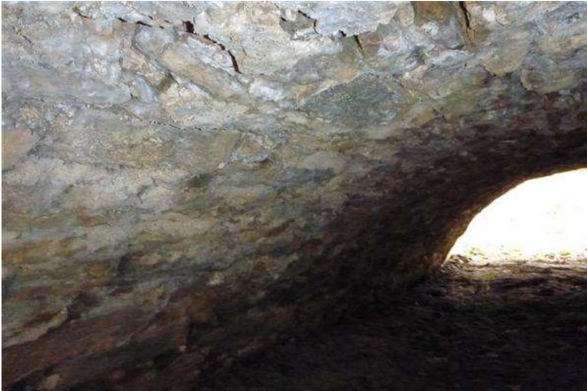
Photo 4 - masonry barrel looking northeast
