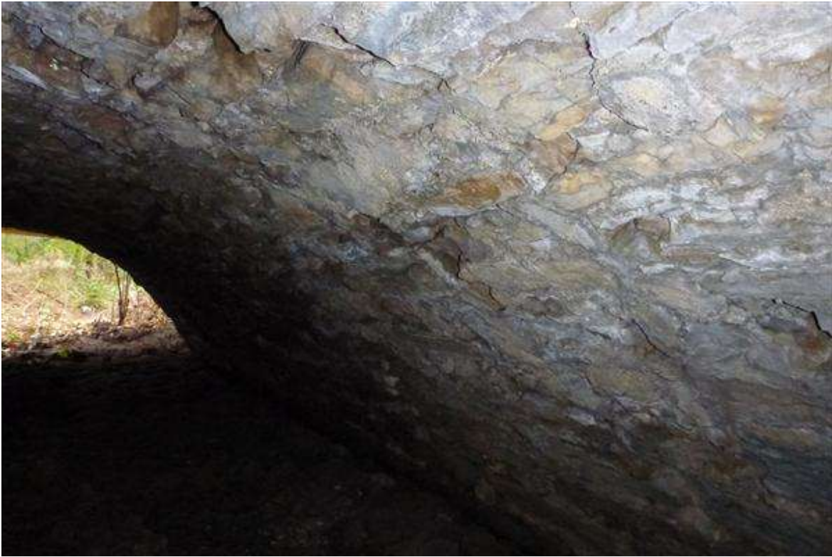
Photo 5 - masonry barrel looking southeast
