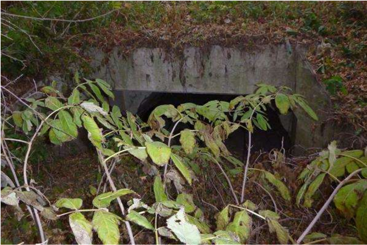
Photo 1 - west headwall looking east
