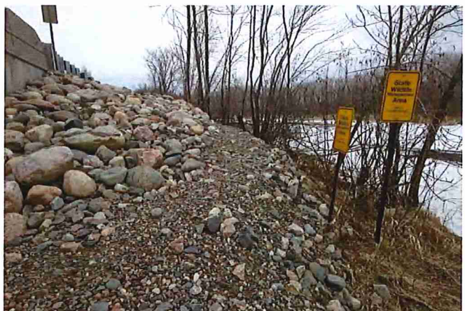
Figure 5. Bench must connect to surrounding topography
