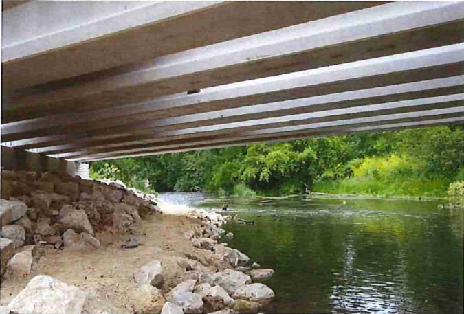
Figure 1. Completed Passage Bench
