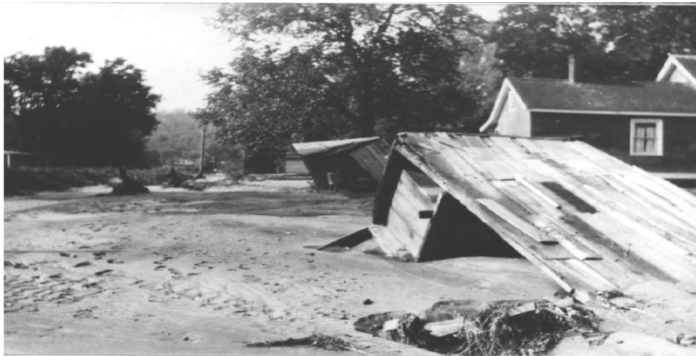
Silt deposition in Afton Village after storm event May 26, 1926 and damaged structures. Source: Afton Historical Museum ( Add image ID # ).
